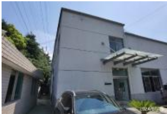
3. 2F office building.jpg
