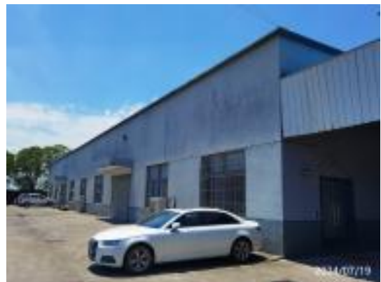
4. 1F production building.jpg
